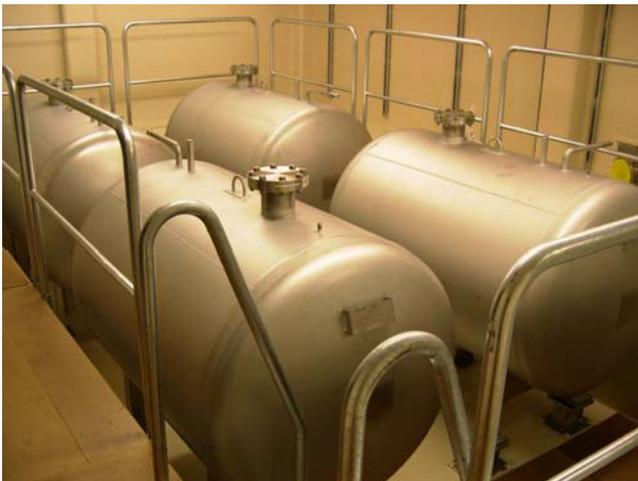
*Figure 6: Storage and leakage tanks for the heavy water circuit (in total 8m<sup>3</sup> ) have been installed.*
