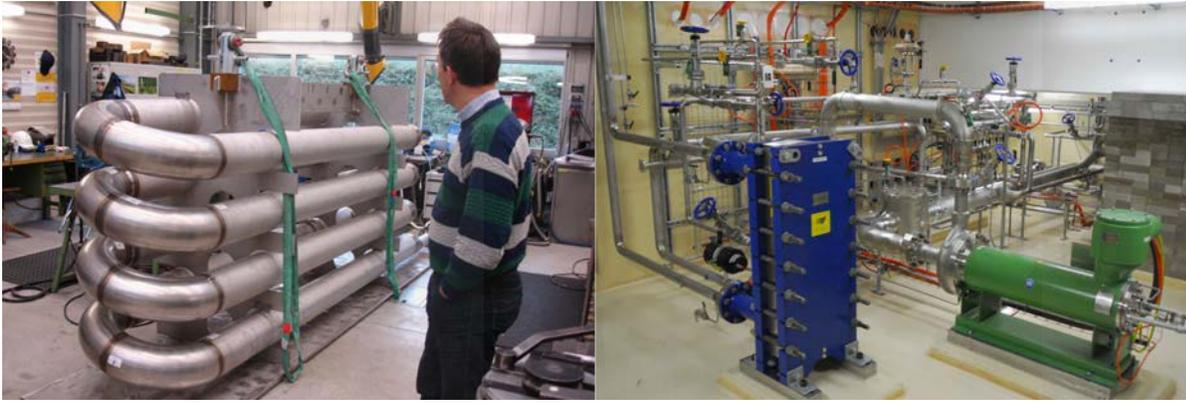
*Figure 7: Delay volume. The heavy water from the spallation target is delayed by about 60 s in order to allow the short-lived radioactive isotopes, created by neutron spallation in the heavy water, to decay before reaching the pumping station. Right: The cooling system.*
