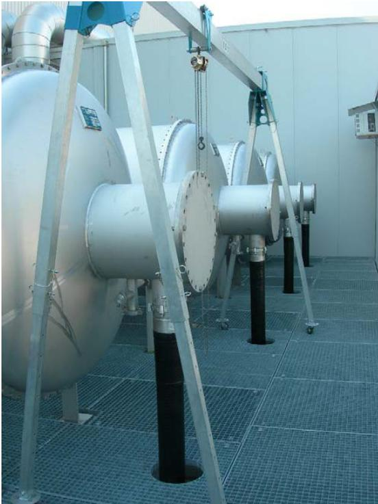
*Figure 8: Storage tanks for the deuterium gas system (in total  $30 \text{ m}^3$ ).*
