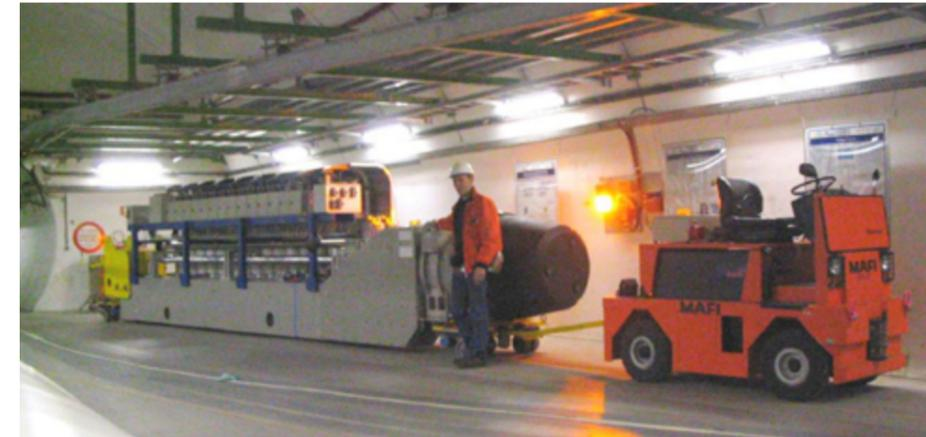
Fig. 5.1.2.1: Example of transport convoy during DFB installation at LHC.
