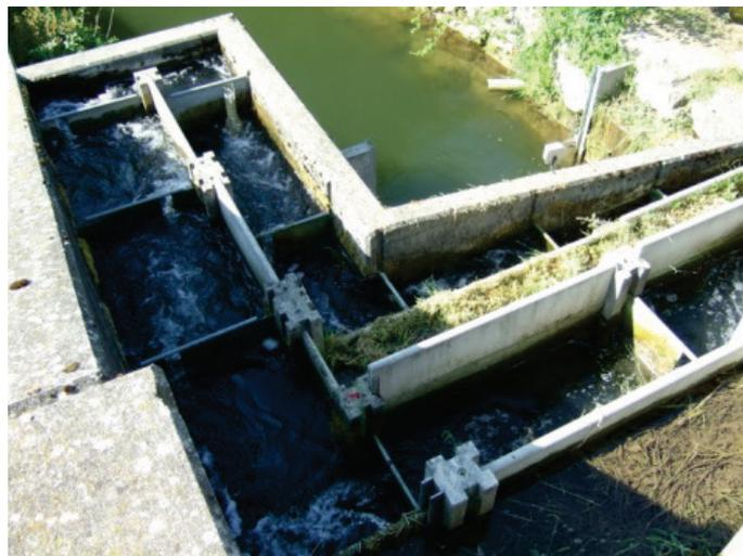
Figure 7.15: Fish ladder at mini hydropower plant Lotzwil. Source: Elaqua Ag
