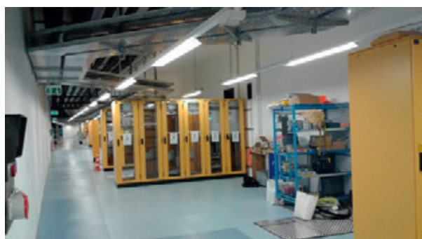
Fig. 5.1.6: Rack gallery in OSFA-UH.020 around z \sim 485\text{m} where the cable trays are deviated to allow the installation of the X band modulator.
