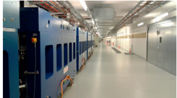
Fig. 1.3.2.3: Sectional view of the SwissFEL Tunnel (z=520 m, looking towards gun), showing the Aramis Undulator line (on the left) and the available space for the Athos line (right).
