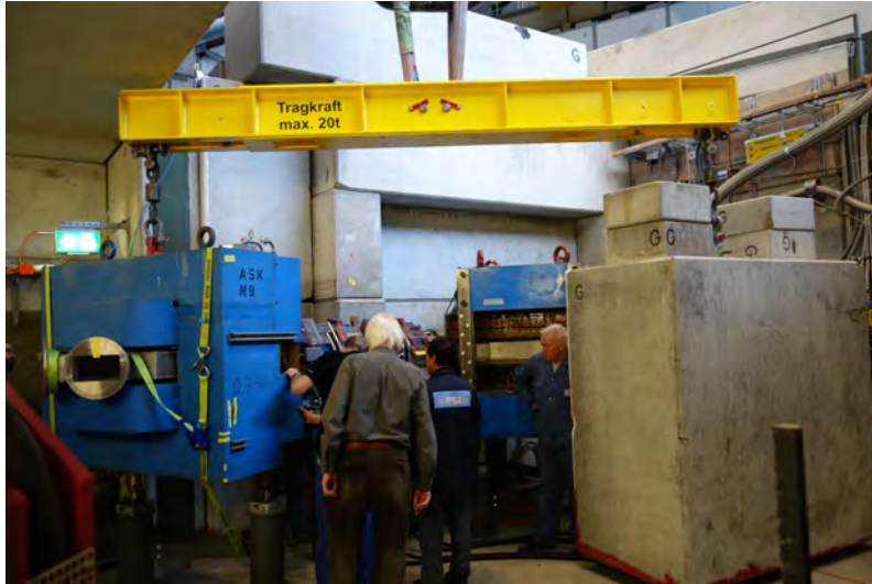
Figure 2.48.: By attaching the ASK dipole magnet to a steel beam with a 10 ton concrete block as a counterweight, the ASK could be accurately placed below the \pi E3 area floor.
