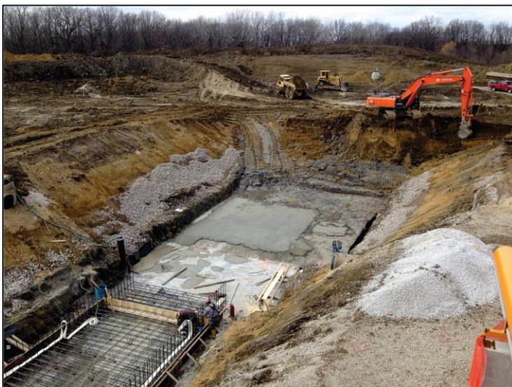
Construction of the mu2e exp hall started at Fermilab
