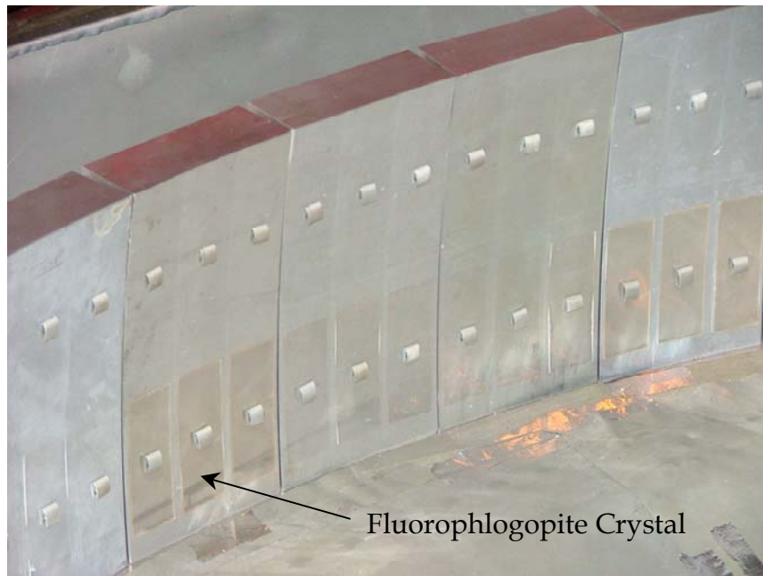
Figure 6. The installation of fluorophlogopite at the half-way stage
