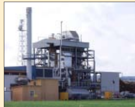
Biomass power plant Güssing (Burgenland, Austria).
