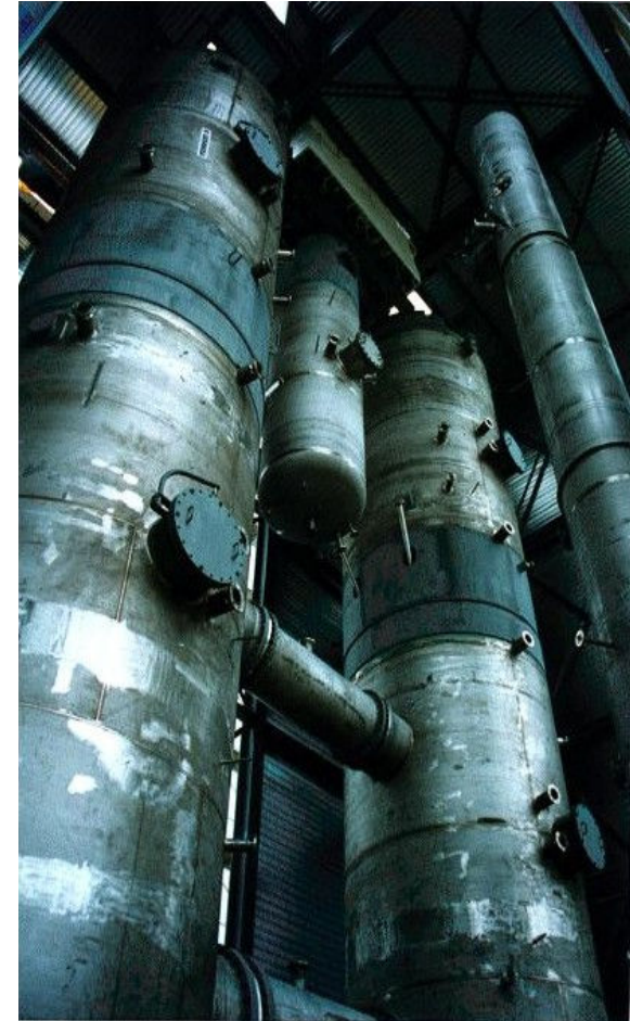
PANDA Vessels ( Construction Phase )
