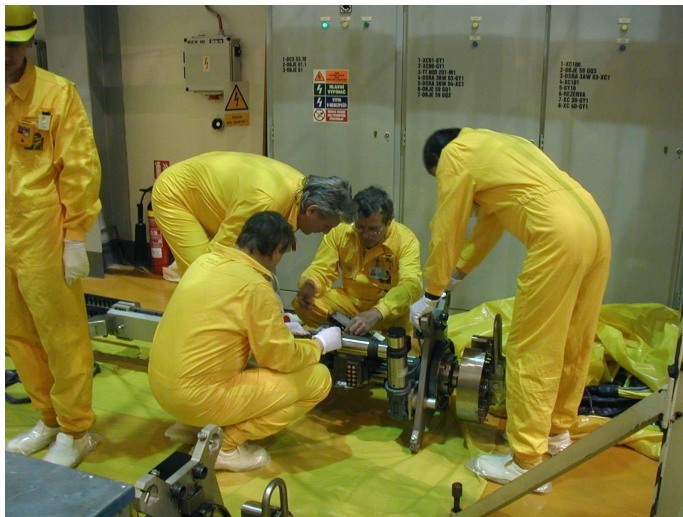
Preparation of manipulator for SG heat-exchanging tubes inspection by eddy currents
