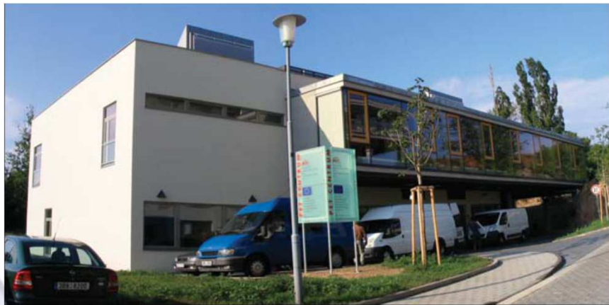
Newly constructed PET Centre in Brno
