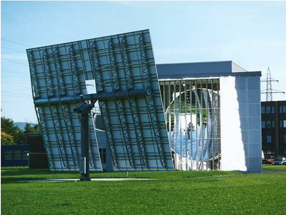
The solar concentrator accumulates 5000 suns
