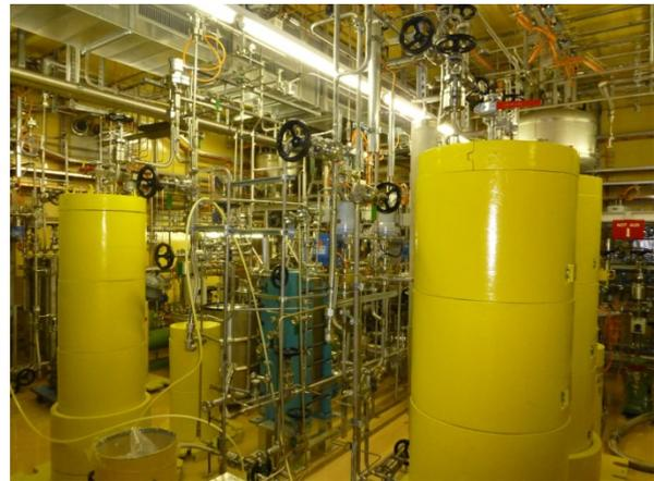
**Fig. 3:** The cooling plant room with shielded ion exchange vessels (front).
