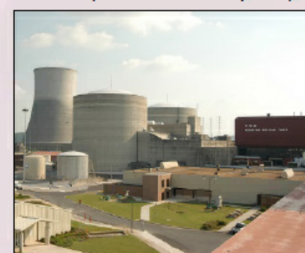
Sequoyah (PWR Ice Condenser Containment in TN)
