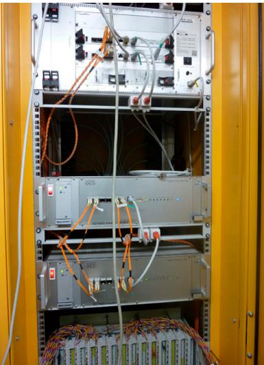
The hardware of the PSI Safety System Adapter installed in the Gantry 3 electronics room. The upper crate holds the two redundant IFC1210® controllers. In the central part of the rack are two Signal Converter Boxes (SCB) that provide connections to external signals from Varian and from PSI. Communication between the IFC210 and the SCBs is handled over fibre optical links (orange cables). The lower part of the rack holds the patch panel with connections to PSI's central safety systems.
