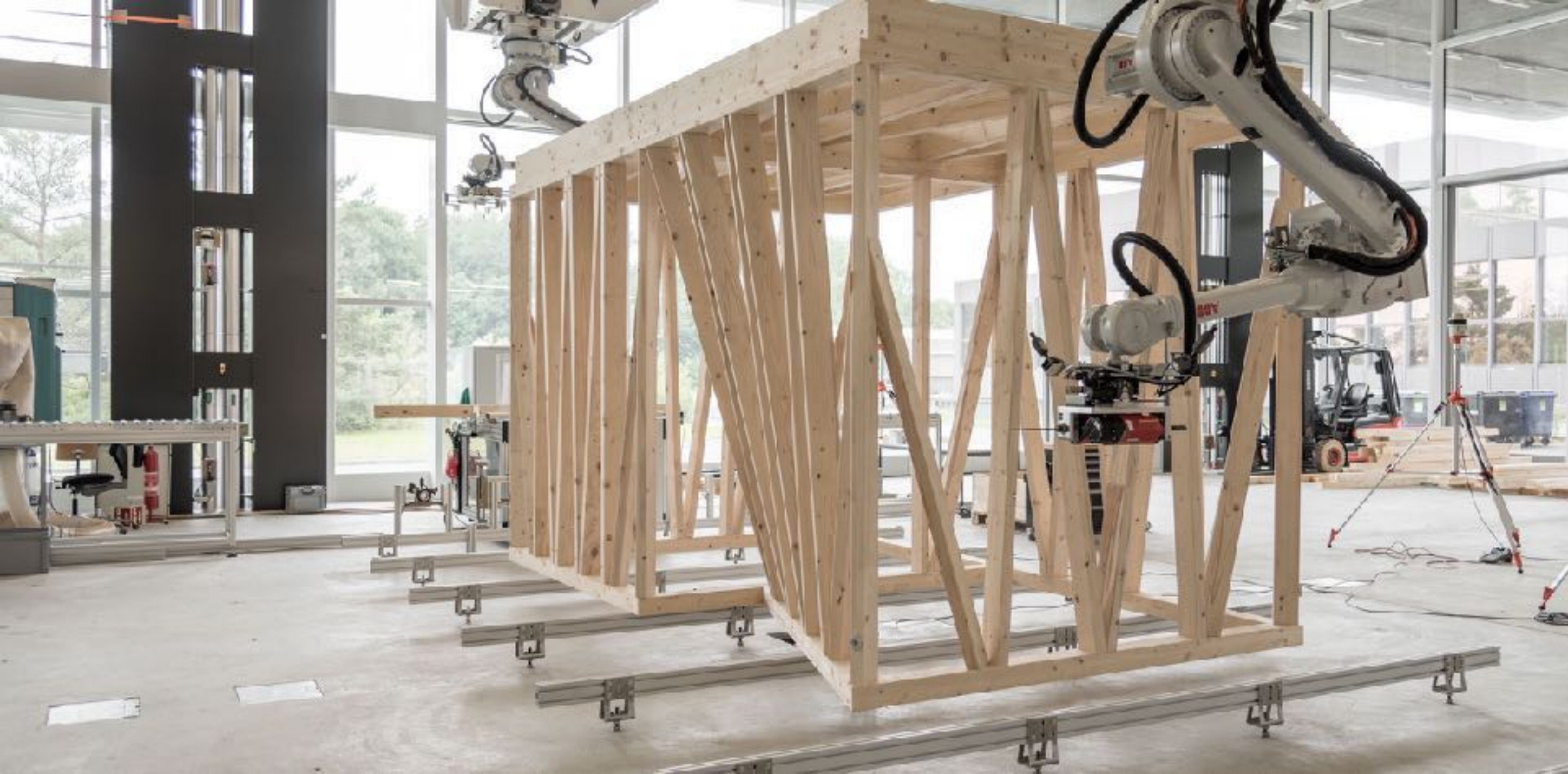
Digital Timber Assembly DFAB HOUSE -NCCR Digital Fabrication
