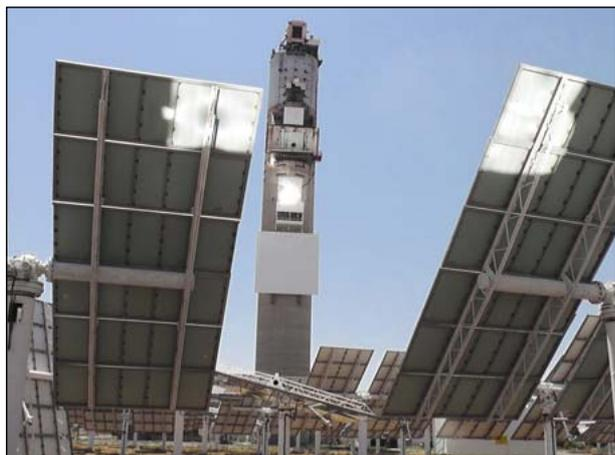
Figure 3: A field of heliostats concentrate solar radiation into the solar gasification reactor located 45m above ground on the solar tower of the Plataforma Solar de Almería, Spain.
