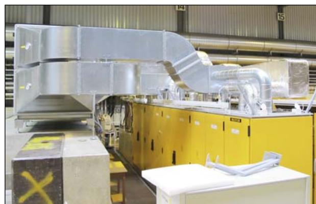
Figure 4: New cooling system for the PROSCAN RF amplifier.
