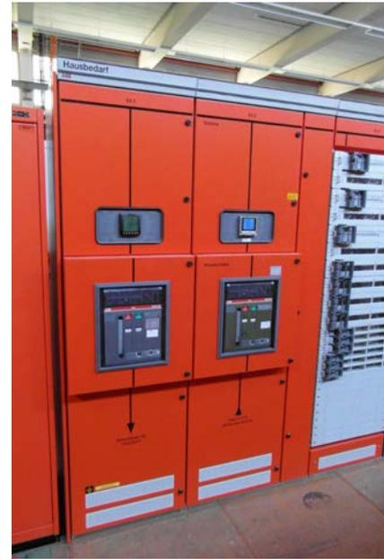
Figure 3: Power cabinet with power breaker, multi-measurement devices and distribution slots.
