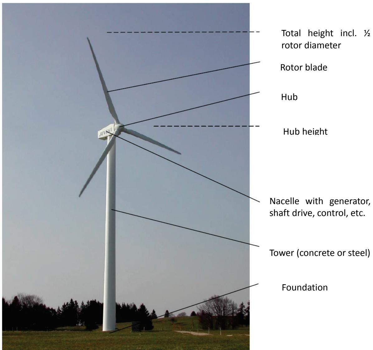
**Figure 8.14: Components of a wind turbine. Adapted from (BFE, BAFU et al. 2004a).**
