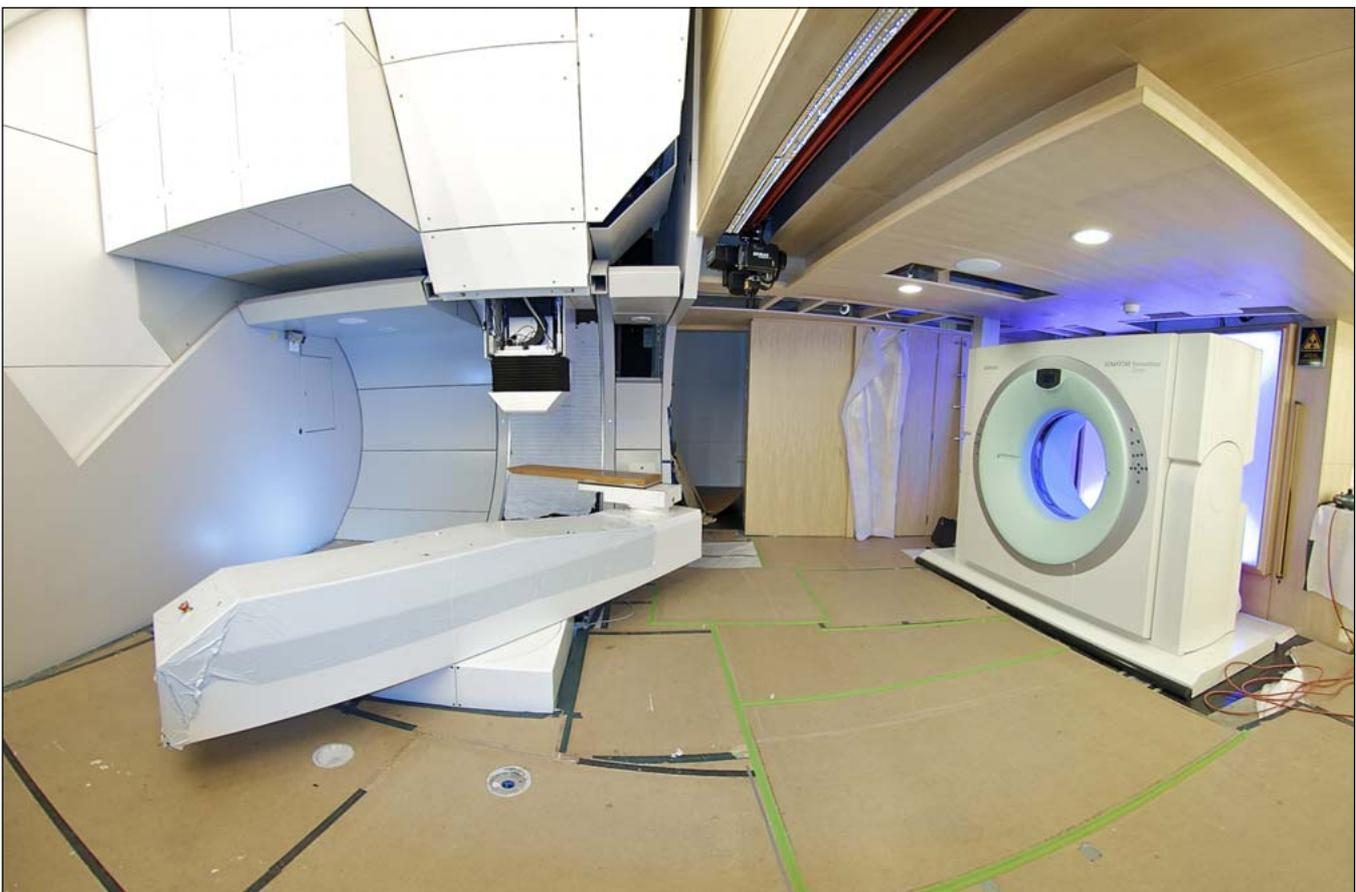
Figure 1: Gantry 2 treatment area nearing completion, with beam nozzle, patient table and sliding CT.
