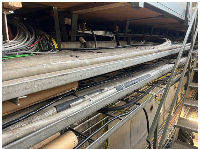
Figure 4.3.2: Filled and partially filled cable trays and a lot of old cables near the PiM1 experimental area.
