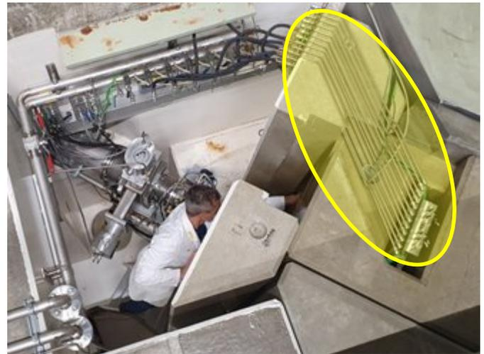
**Figure 2:** top view of the region before the beam stopper BX2 (to the right). The yellow area denotes the cooling pipes, which have a high leverage on the ceramic feedthroughs if detached. The colleague is working on the leaking flange.
