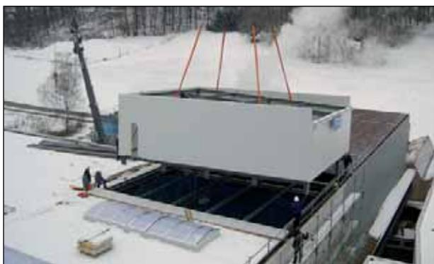
Figure 2: **Positioning of the air conditioning housing on the roof of the experimental area.**
