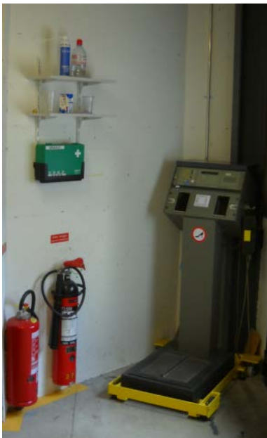
Fig.4: Radiation monitor. On the top left the shelf where temporary storage of drinking bottles is allowed.
