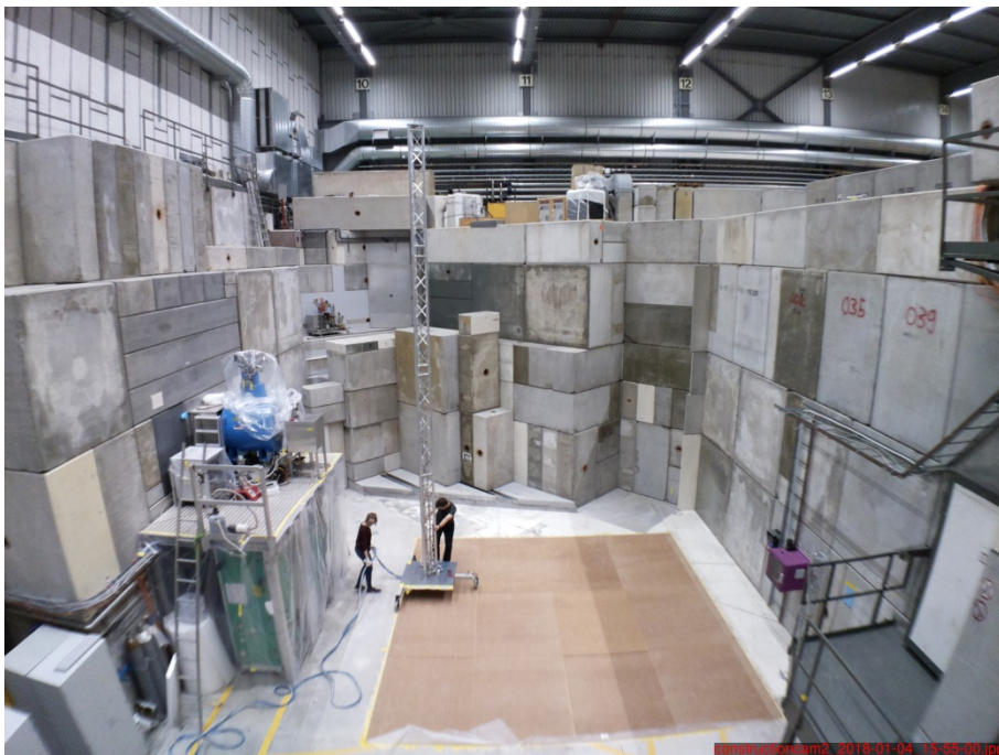
Fig.17: empty area south with SC magnet
