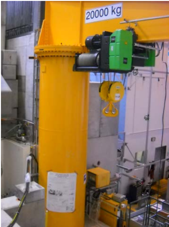
Fig. 22: Crane serving partially area West and area South
