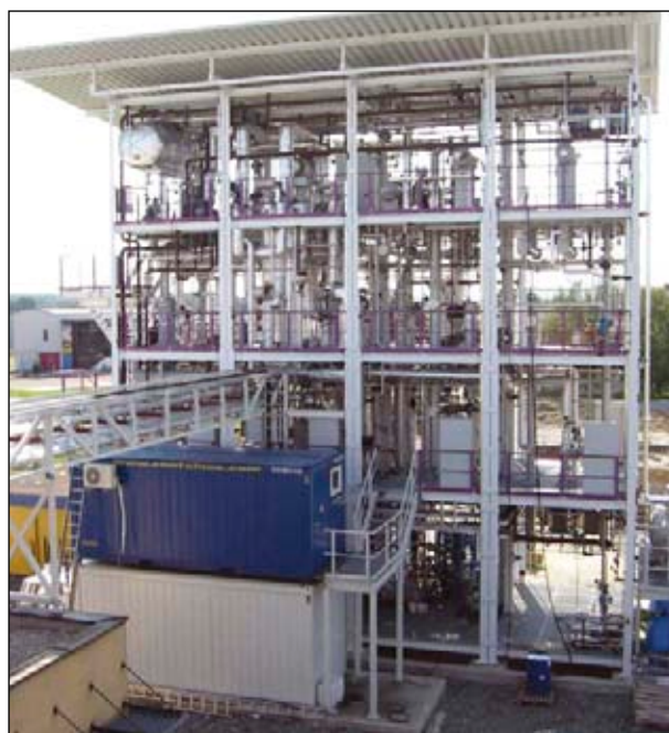
Figure 1: Biomass power plant at Güssing, Austria.
