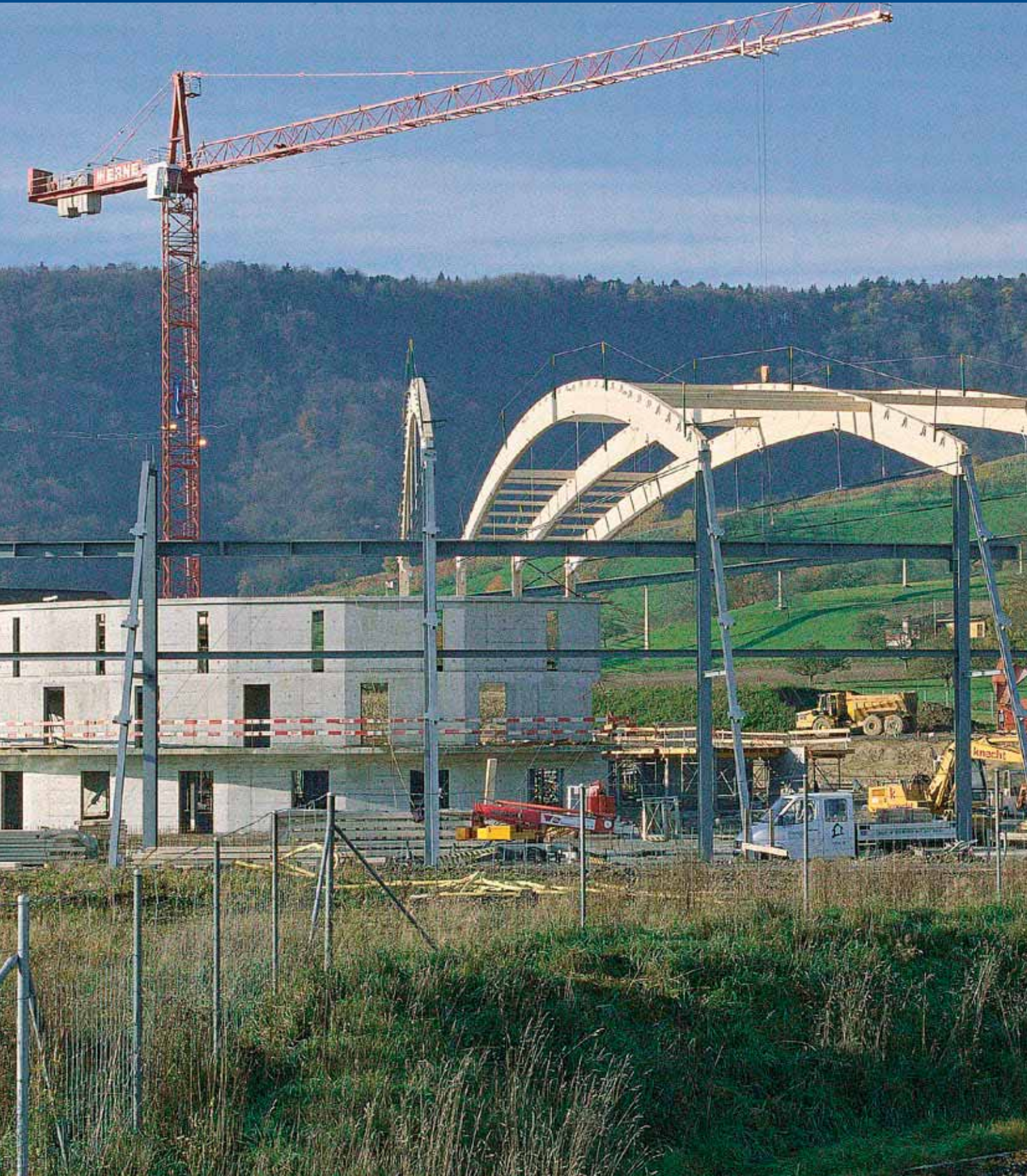
The beginnings of construction in 1998: the SLS is taking shape.
